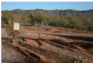
Old parking areas, re-contoured
